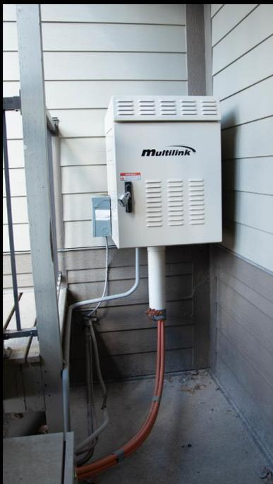
At the Firehall A Multilink 12RU Cabinet w 72 circuit ODF and 72 Gigabit SFP Switch Ports With 30 hour power Support \$11,900
